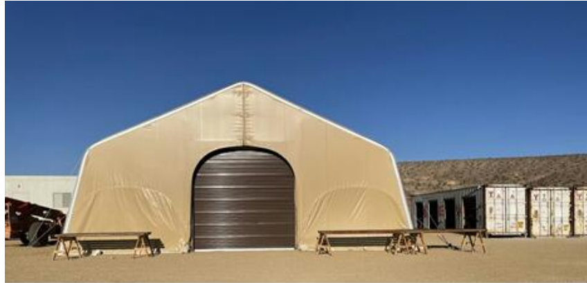
Figure 8-4: Core Shed and Quick Log Station
